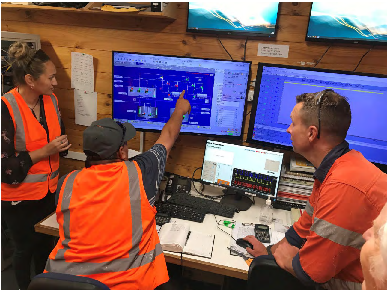
Mayor Faylene Tunui views the upgrades of the Three Waters plant including the wastewater treatment facility.
