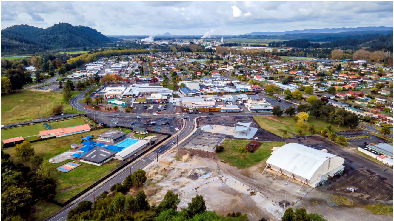
The Maurie Kjar Aquatic Centre and the Ron Hardie Recreation Centre (right foreground).
