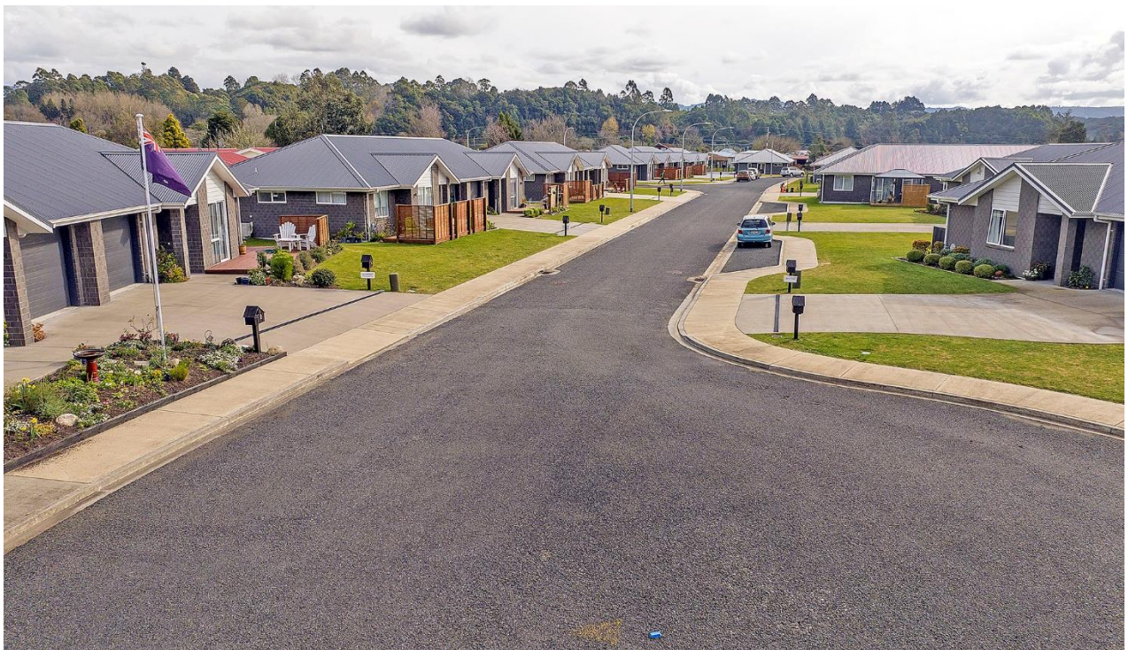
Porritt Glade Lifestyle Village – a finalist in the Taituarā Local Government New Zealand Awards In the Beca Placemaking Category.
