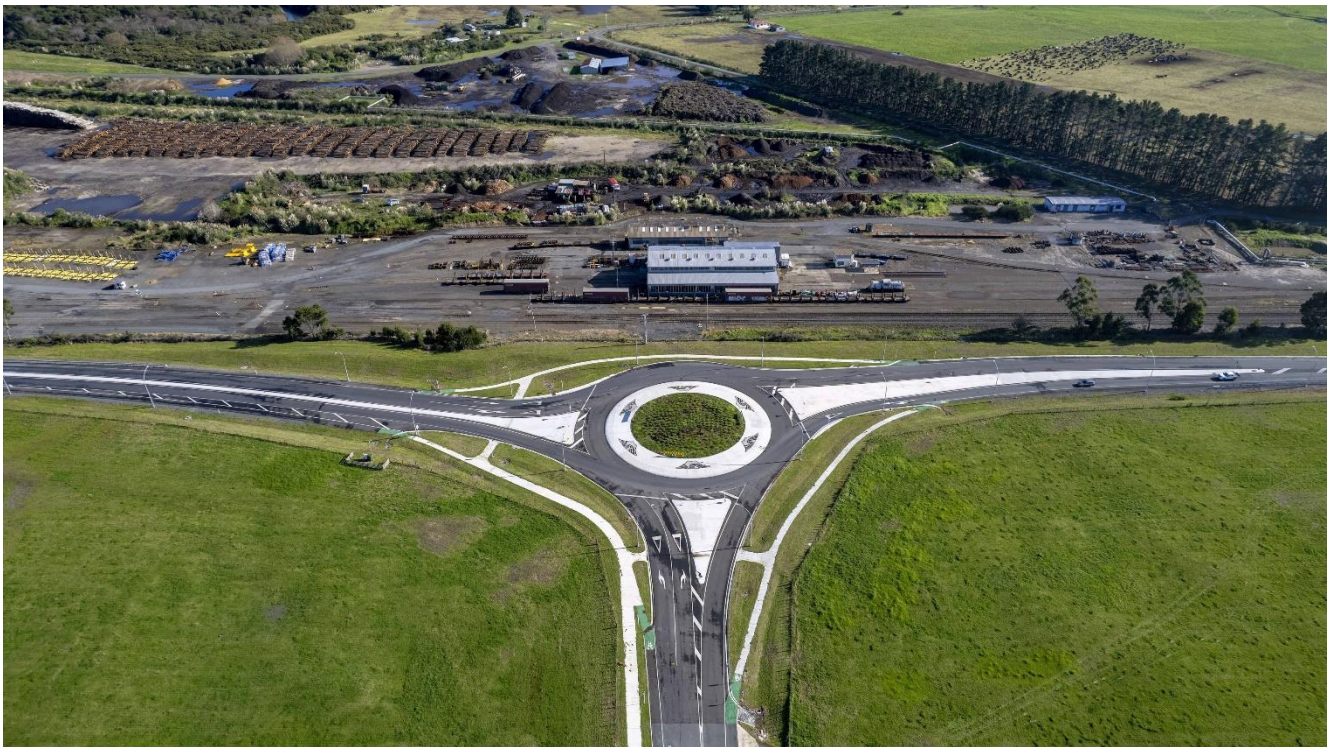
The roundabout on State Highway 34 developed for entry into the Putauaki Trust Industrial Zone.
