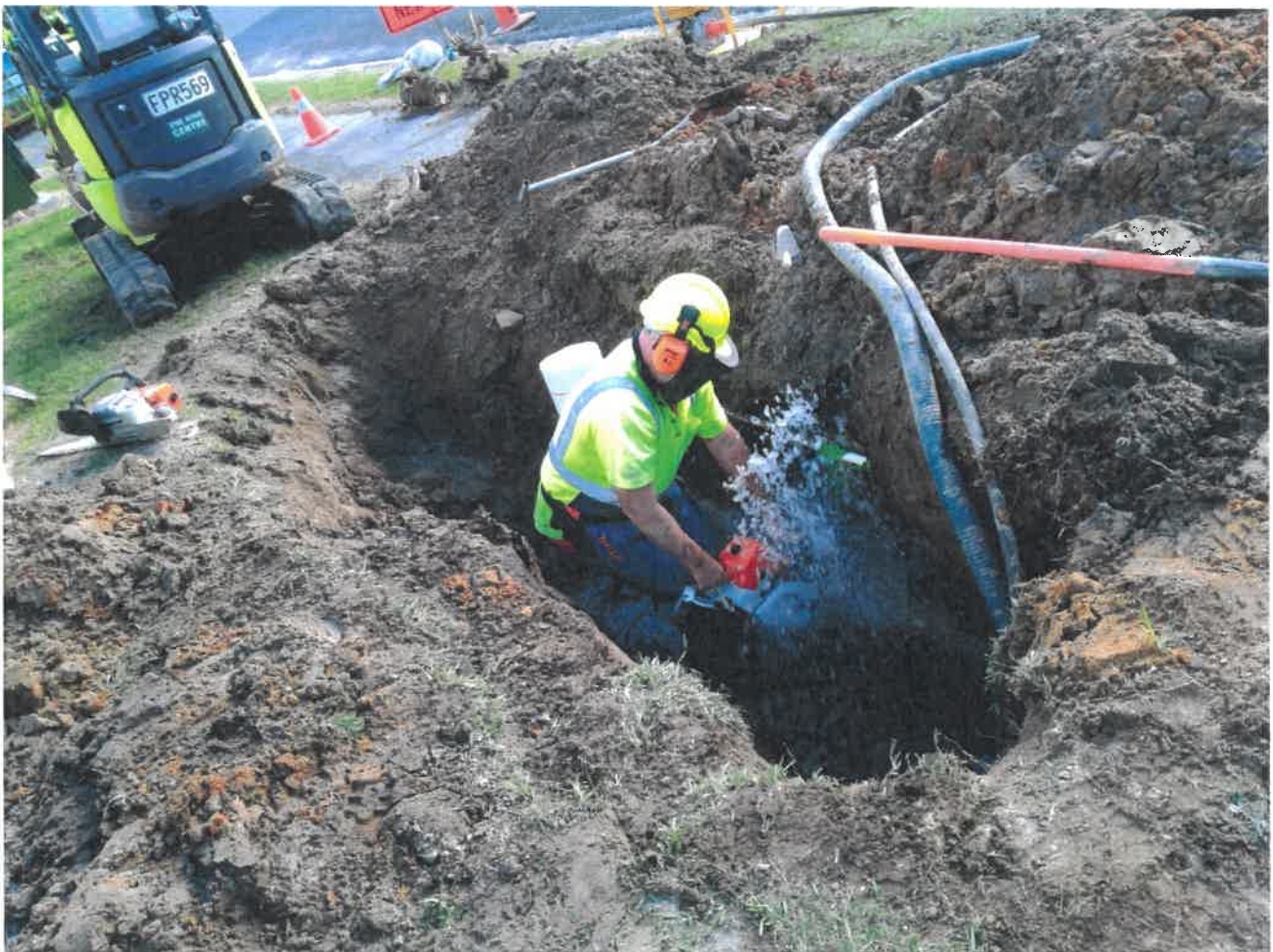
Kawerau's drinking water reticulation (pipe) replacement project.
