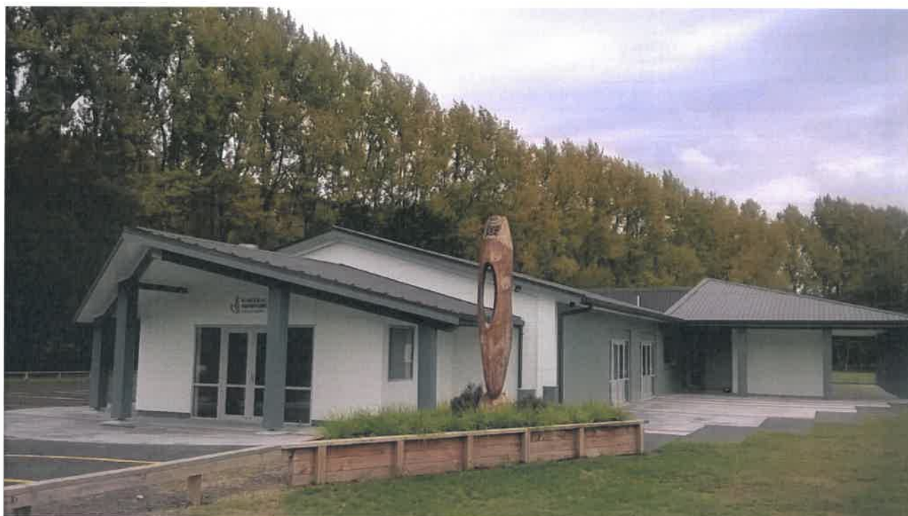
Firmin Lodge – a meeting and 60-bed dormitory style accommodation facility in Kawerau.
