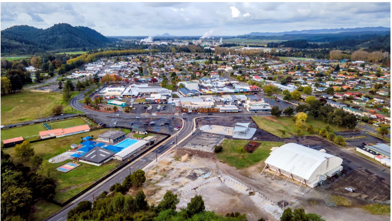
The Maurie Kjar Aquatic Centre and the Ron Hardie Recreation Centre (right foreground).
