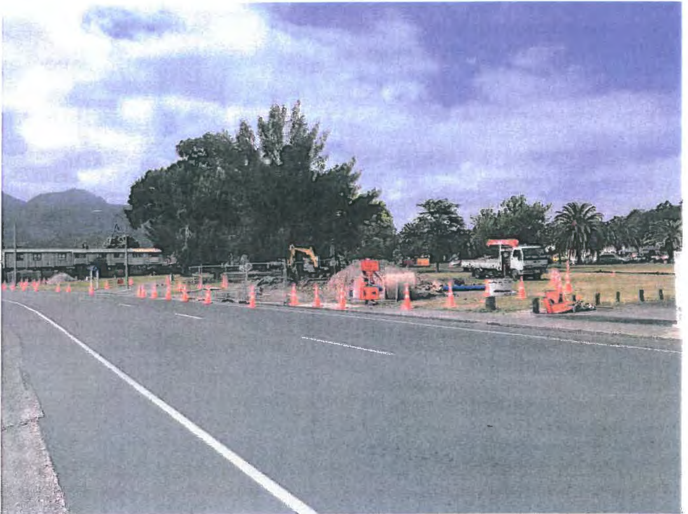
PIPEWORK RENEWAL ALONG PLUNKET STREET
