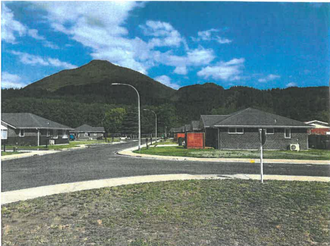
SOME OF THE UNITS COMPLETED DOWN PIRIPIRI CRES
