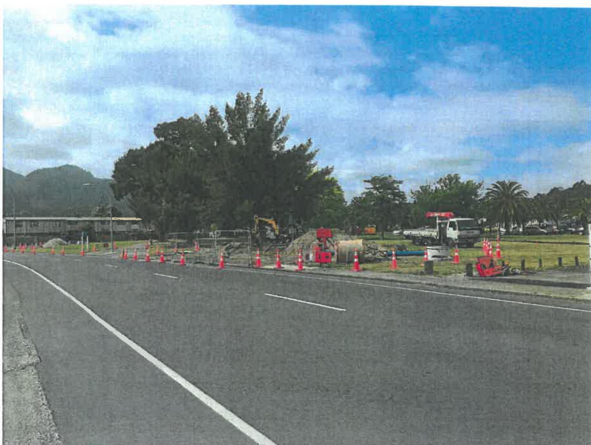
PIPEWORK RENEWAL ALONG PLUNKET STREET
