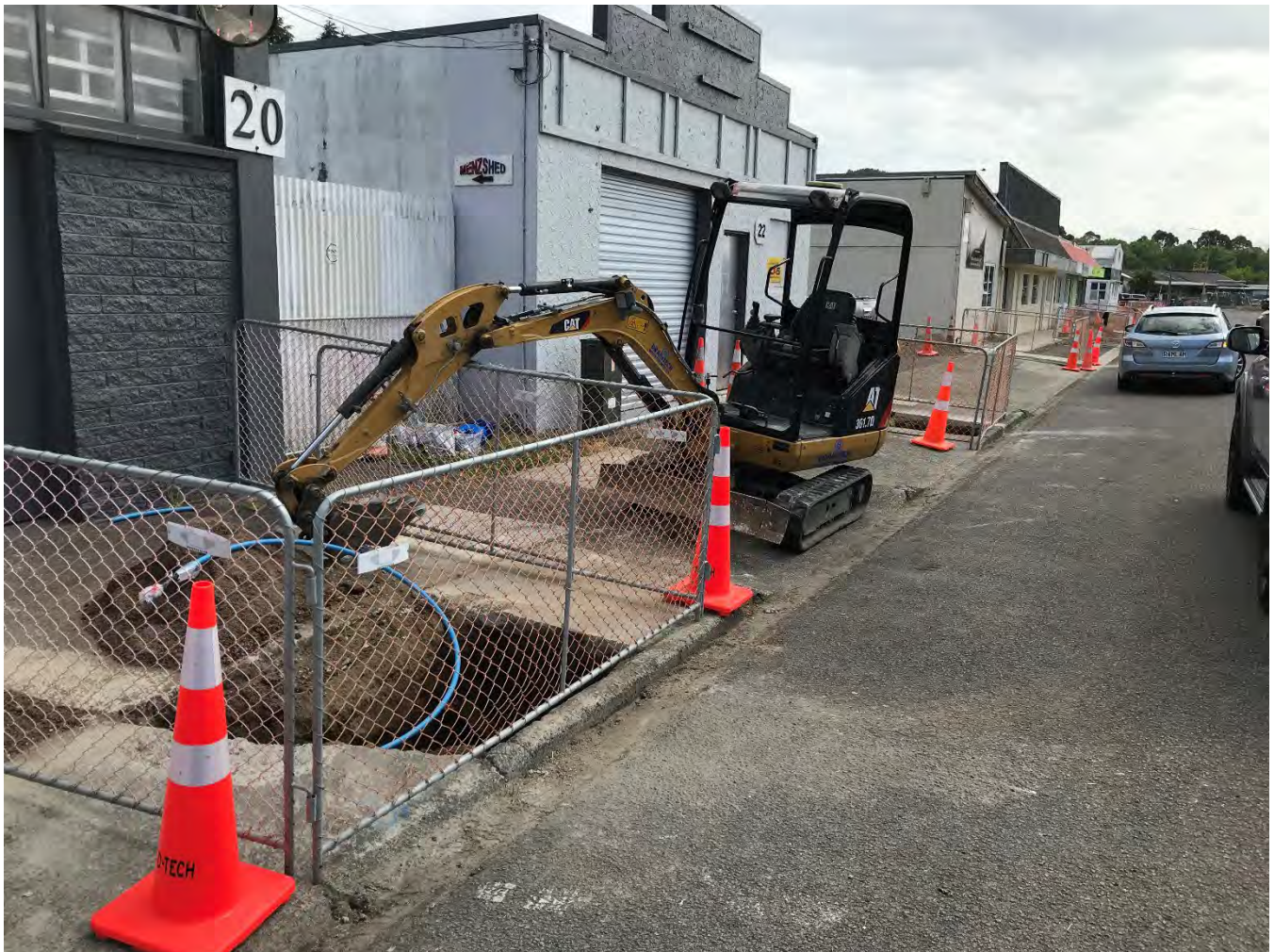
Pipework replacement in Liverpool Street in Kawerau undertaken by Council.
