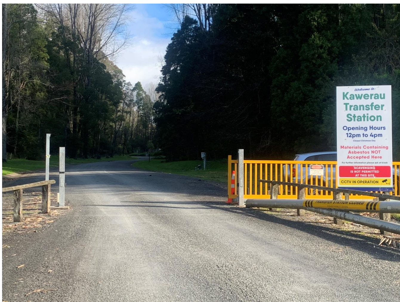
Entrance to Kawerau Transfer Station comprising refuse, greenwaste and recycling operations.
