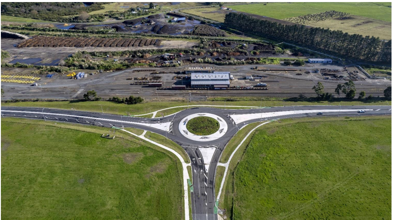
The roundabout on State Highway 34 developed for entry into the Putauaki Trust Industrial Zone.
