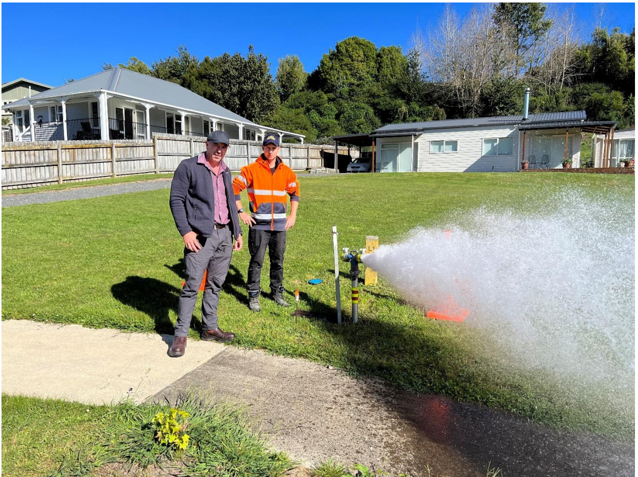
Group Manager, Operations and Service Riaan Nel and Three Waters Team Leader Glen Penny flushing potable (drinking) water lines.
