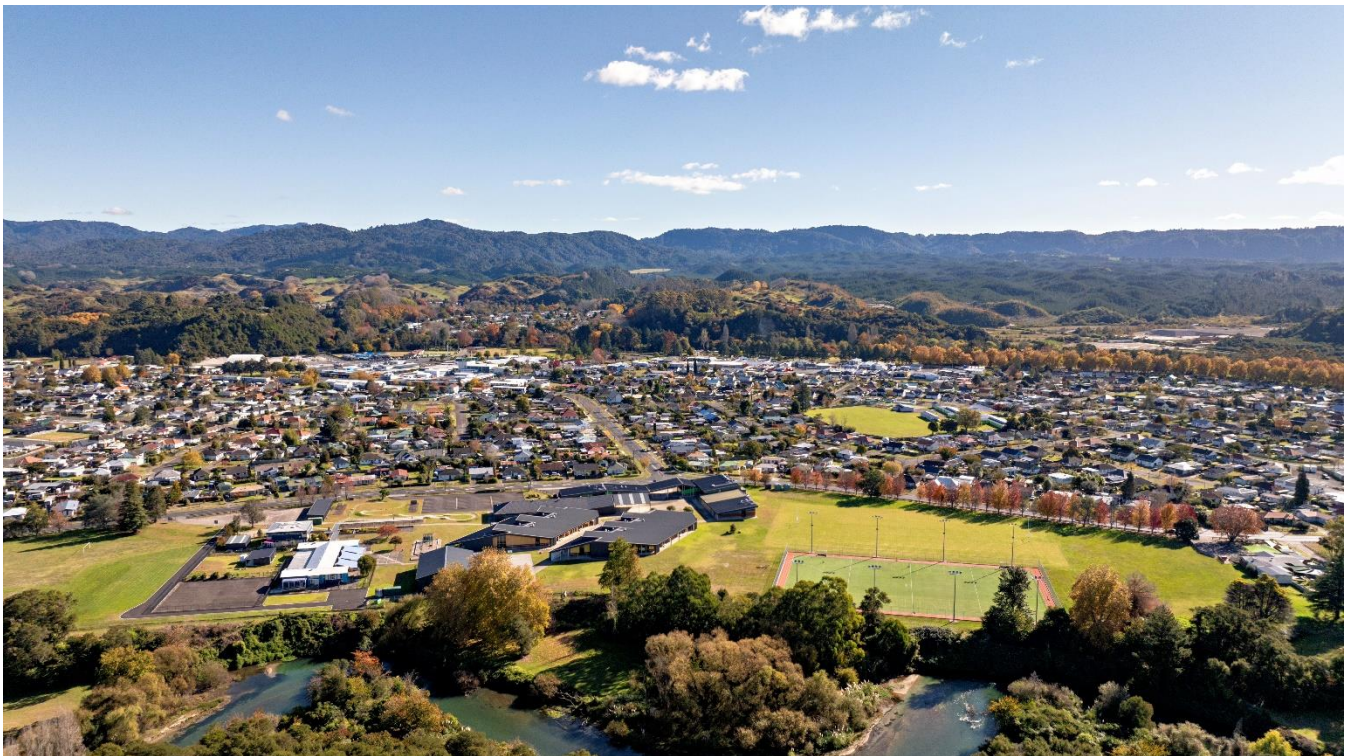
Renewals of drinking water reticulation continue throughout the district continue as per the Long Term Plan 2021-2031.
