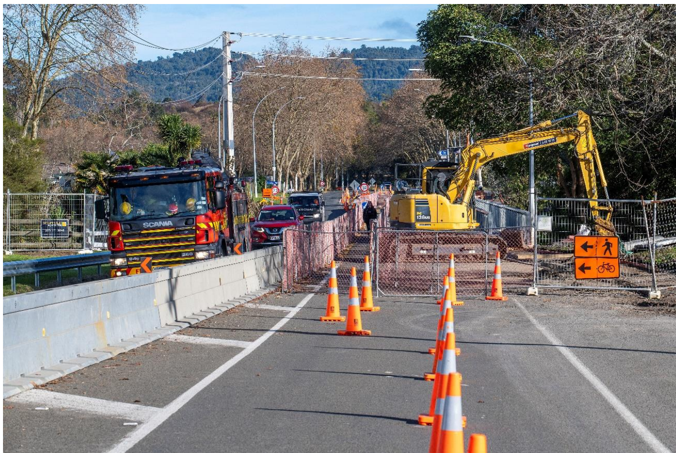
Road works being completed along Tamarangi Drive and State Highway 34.
